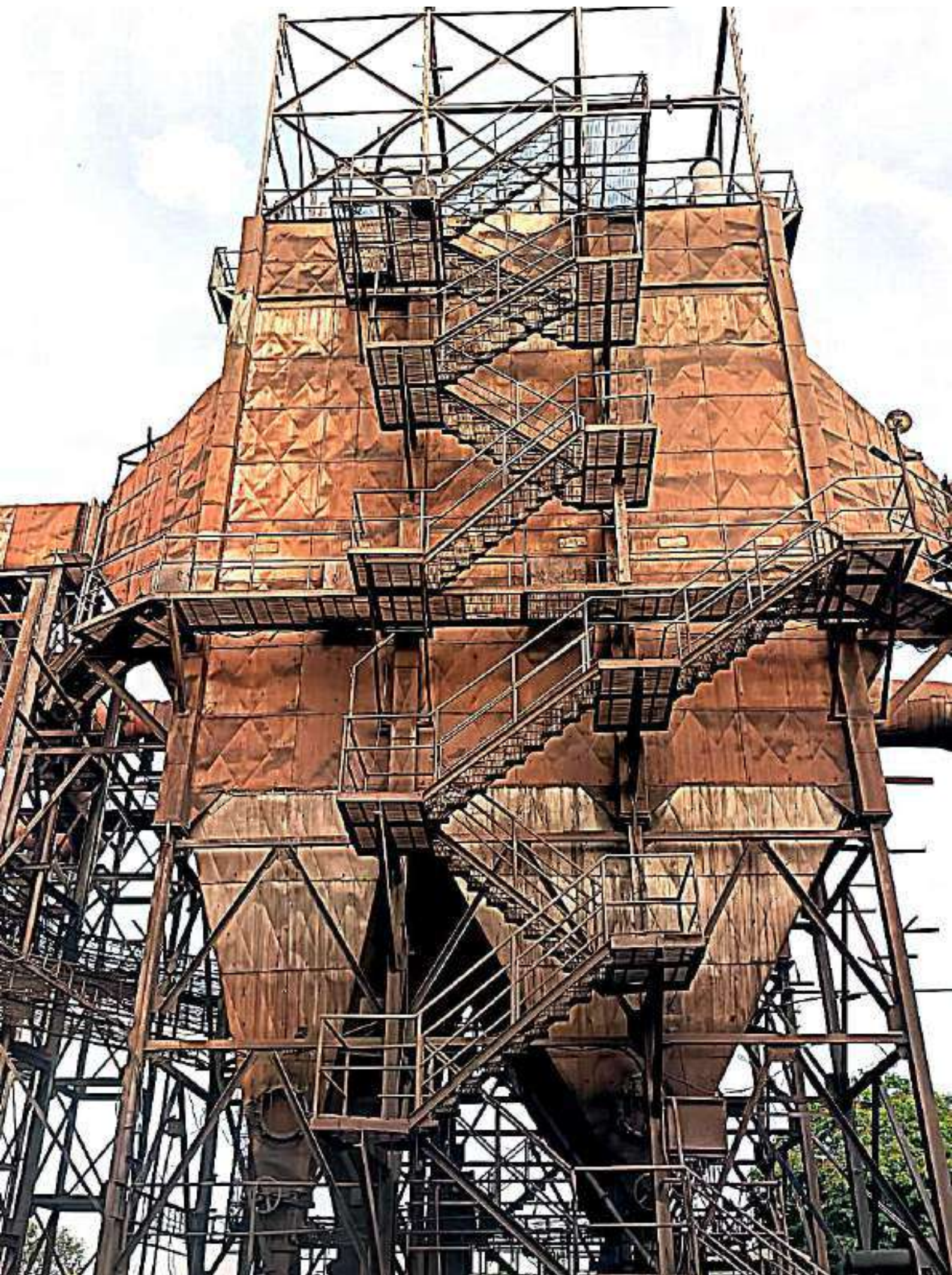
(a) ESP 2 Nos. with common stack
